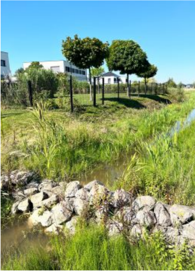
Pierrier, source : Cabinet CHEROUTRE, 2023
